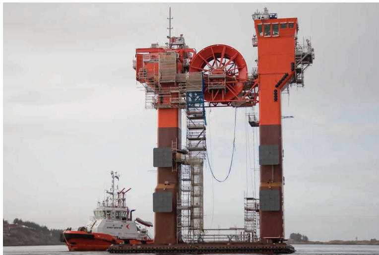
Getting ready for inclination tests.
